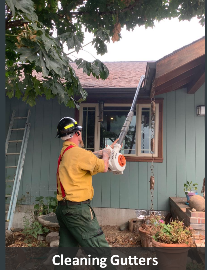
Removing Combustible Debris
